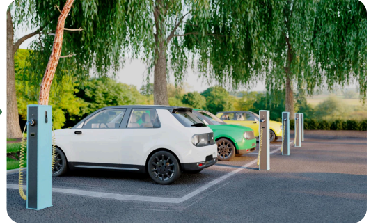
Workplace EV Charging
