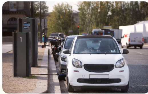
Public EV Charging
